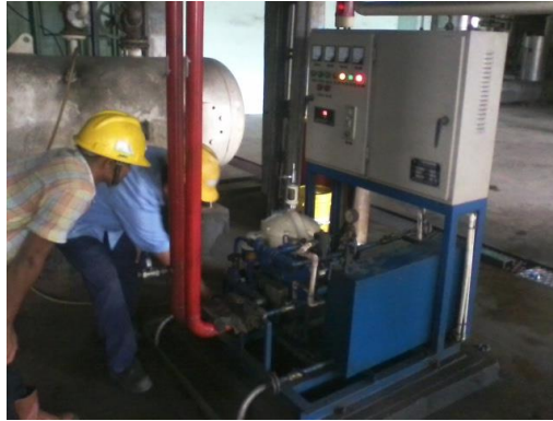
Gambar 3. 6 Oil Separator Cleaning
