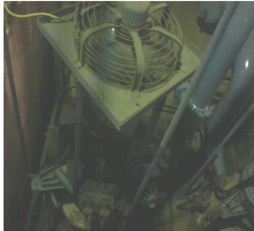
Gambar 2.34 Condensate Extraction Pump
